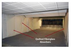
Make sure all drywall and soundproofing is rated as flameretardant. And, be careful about building a wall on top of a crevice in the floor. This can become a place where flammable dust accumulates.
